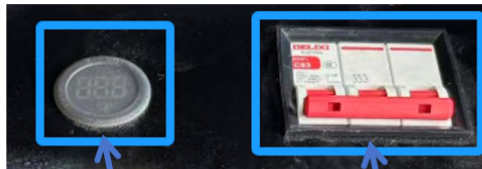
Battery voltage display
